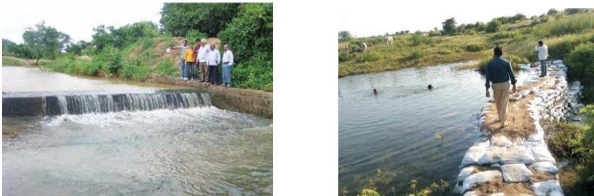
Figure: Low cost sandbag checkdams at Singhbhom
